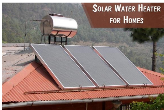
A typical solar water heater is installed on the rooftop.
